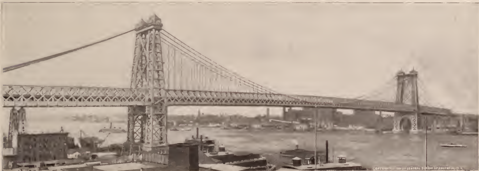
THE NEW EAST RIVER BRIDGE.
